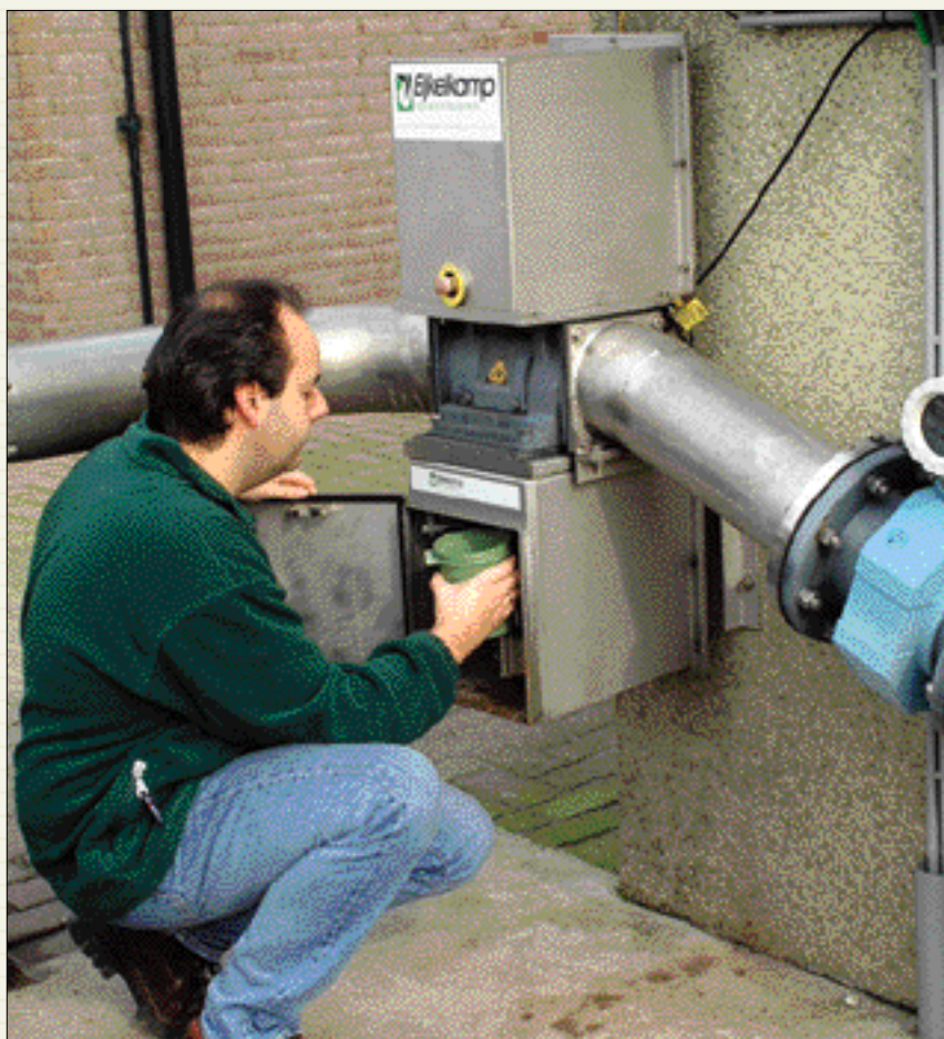
Stationary automatic fraud-proof sampling system
