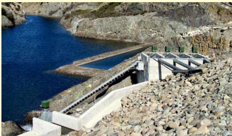
*Each of the five green enclosures shown in the photograph houses a 6541B encoder which measures the water level in a stilling-well coupled to the associated flume. [Photo: Lindsay Anderson, ECS]*
