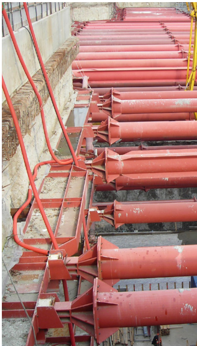
Struts in urban excavation for new Rome metro station
