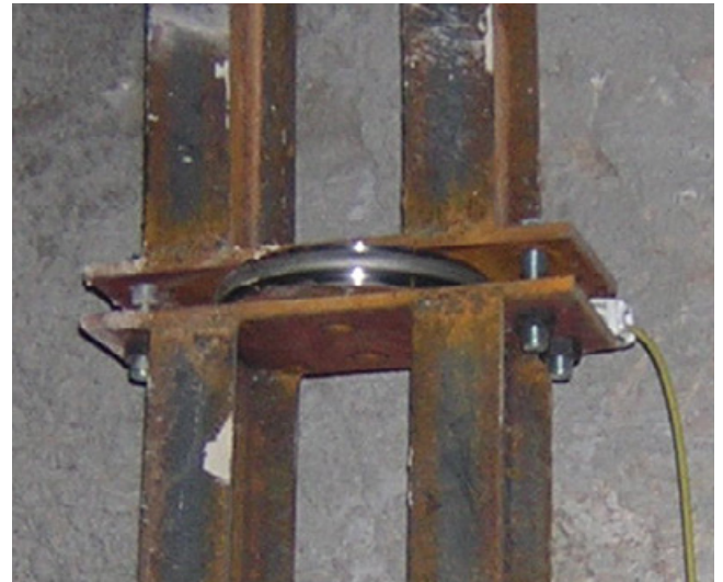
Load cell between two steel lining sections
