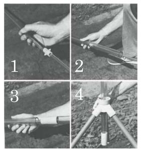
Fig. 35 - Adding Air Tubes and Support Tube Extensions.
