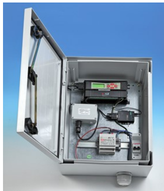
IP66 enclosure for fix monitoring applications.
